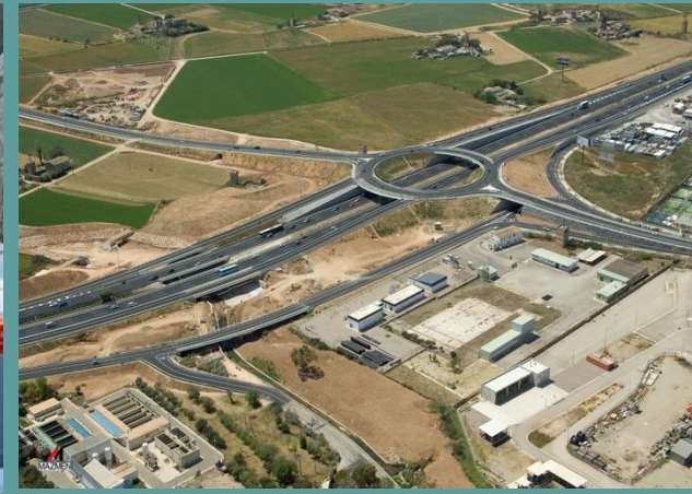
Continual program of widening & construction of highways across the island
