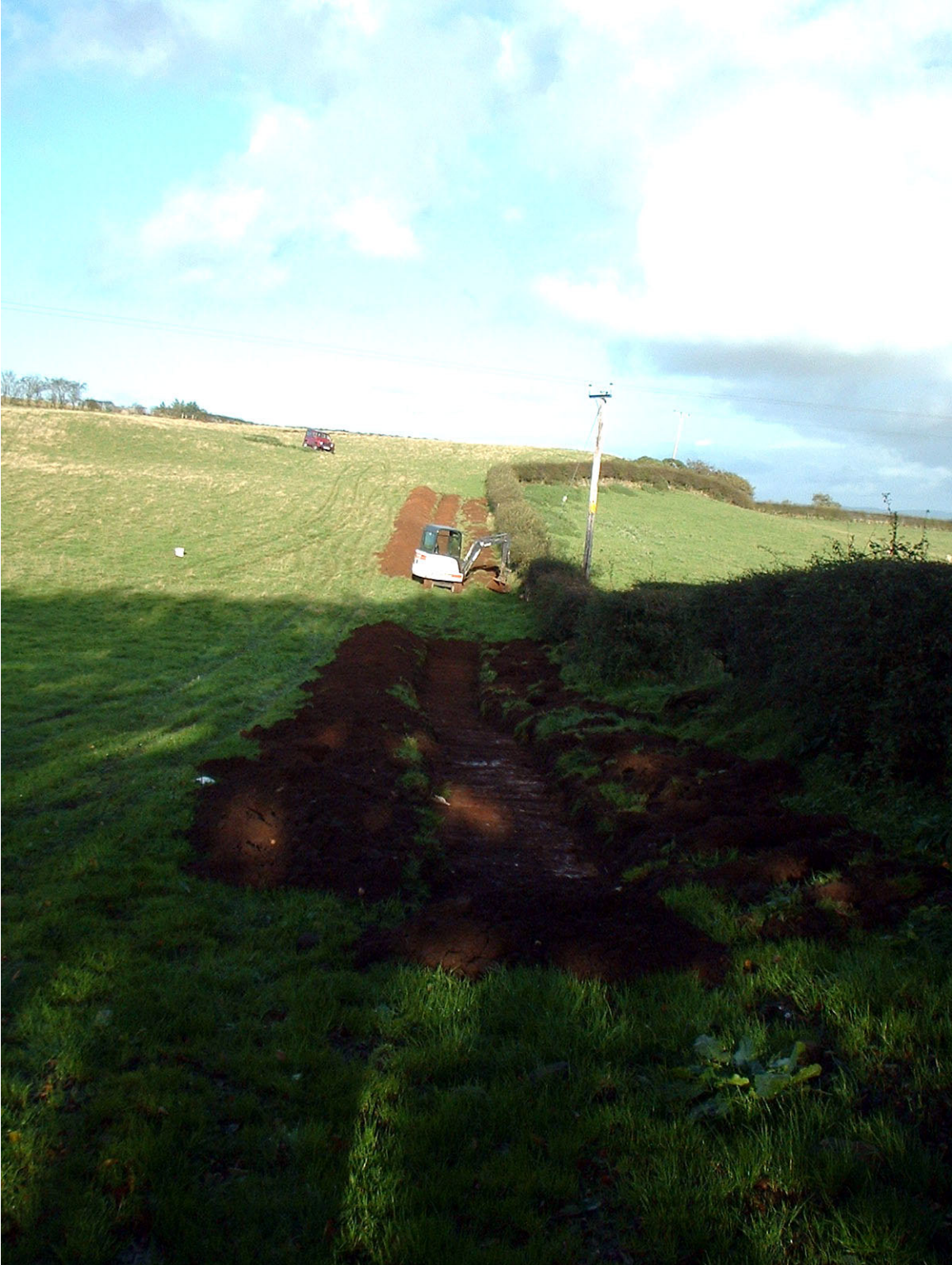
Photo 5: Trench 5 after excavation
