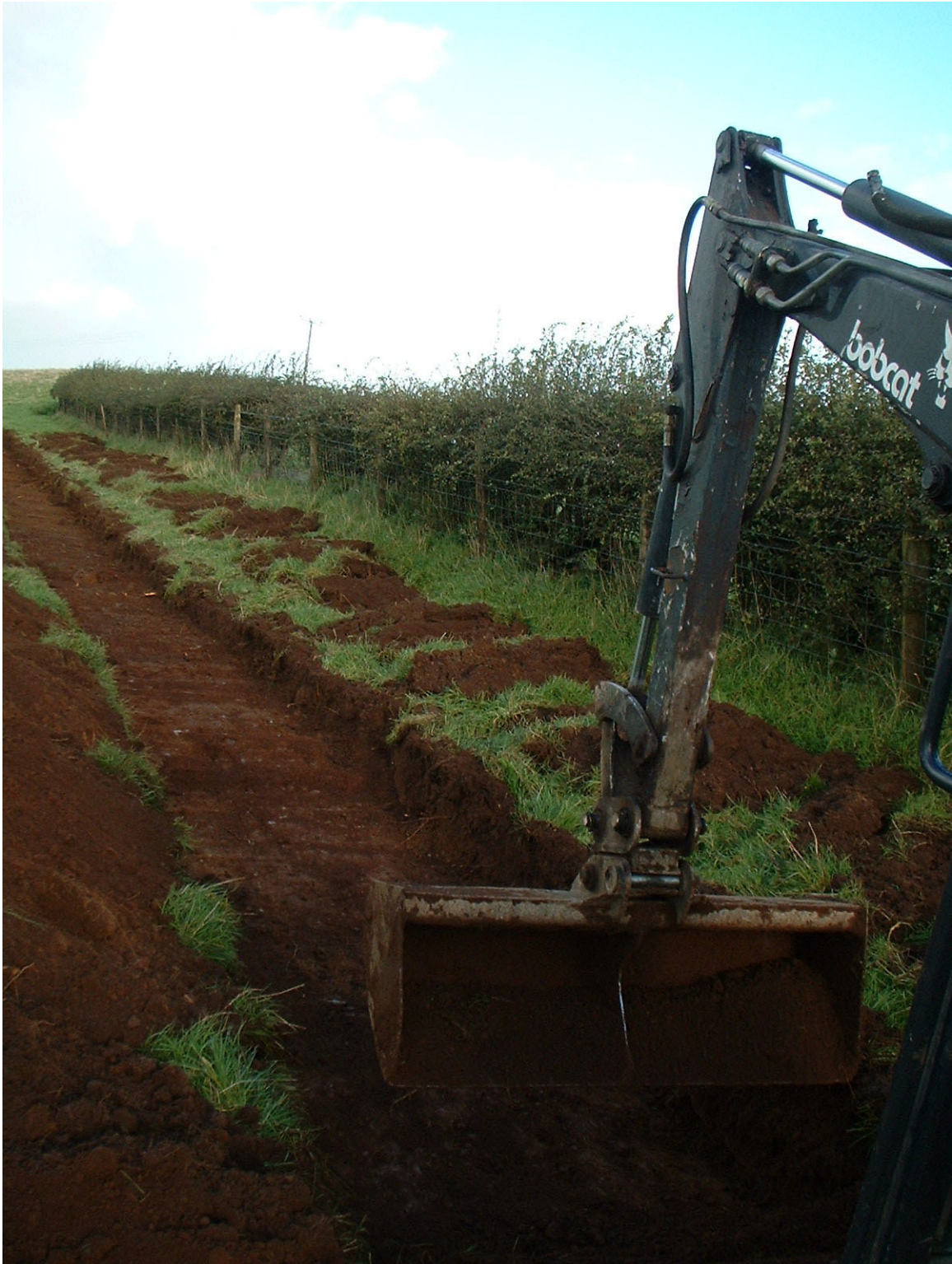
Photo 6: Excavation of Trench 5 showing utilization of toothless “sheugh” bucket
