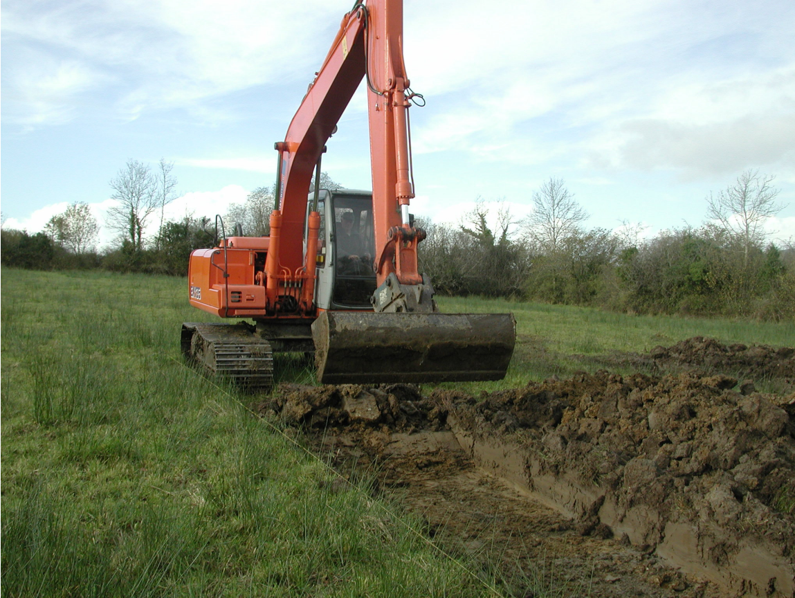
Photo 6: Excavation of Trench 5 showing utilization of toothless “sheugh” bucket.
