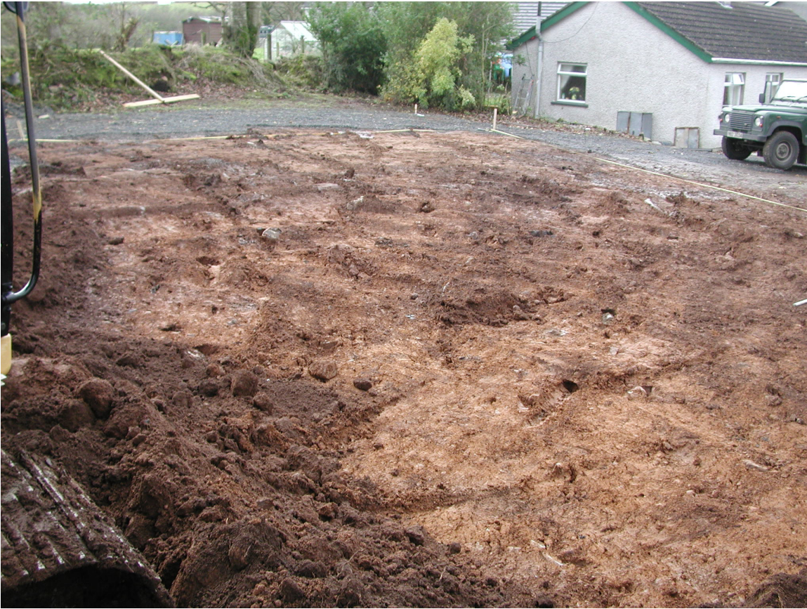
Photo 1: Re-stripped development site from north-east
