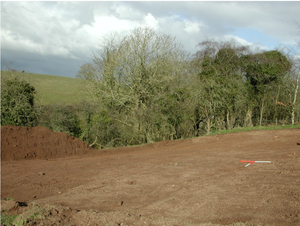
Plate 4: View of northern part of site, in vicinity of Point C, after excavation to subsoil level (C303).
