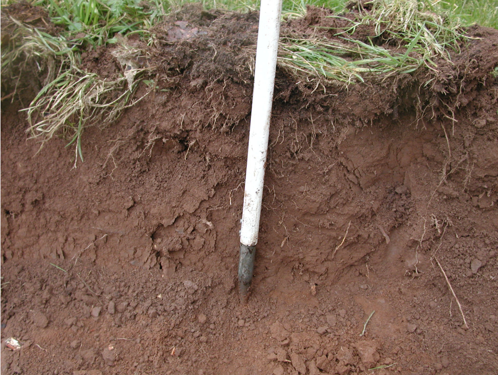
Plate 5: View of section at Point A after excavation to subsoil level (C103).
