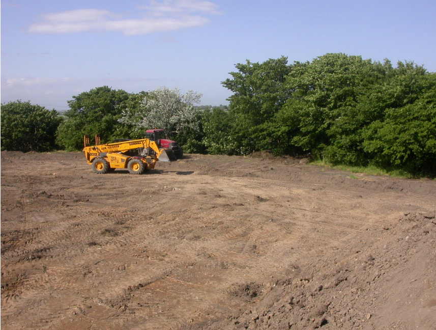
Plate 7: View of topsoil stripped area from south-west.
