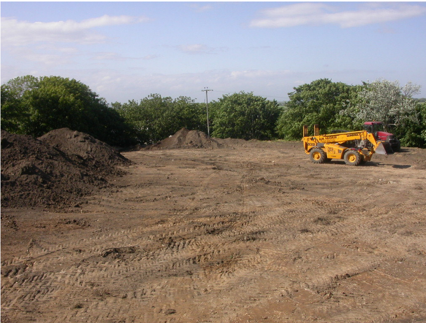
Plate 6: View of topsoil stripped area from south-west.
