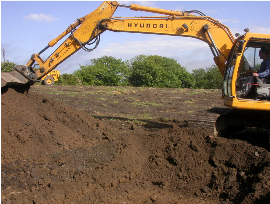
Plate 1: Overall view of site from south-east prior to removal of topsoil.
