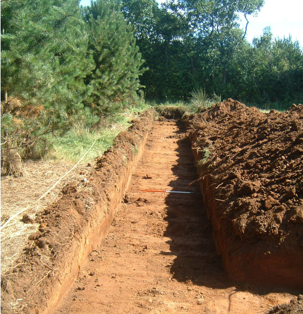
Plate 4. Trench 1 at completion of excavation (Facing north-east)
