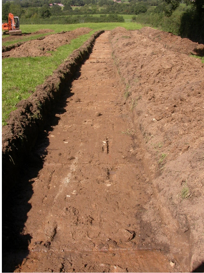
Plate Seven: Trench Two following excavation to subsoil (Context No. 203), looking north-west
