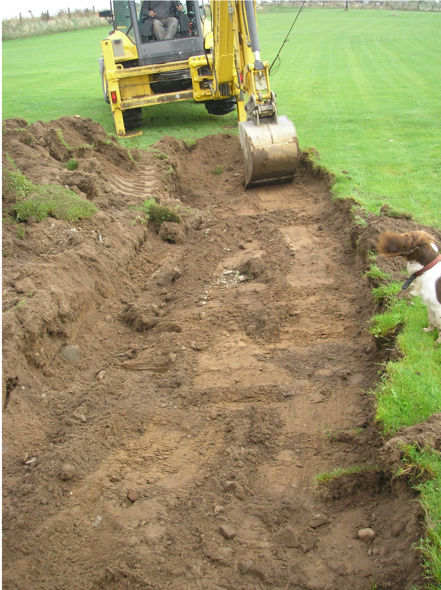
Plate 1: Excavation of Trench 1, looking east.
