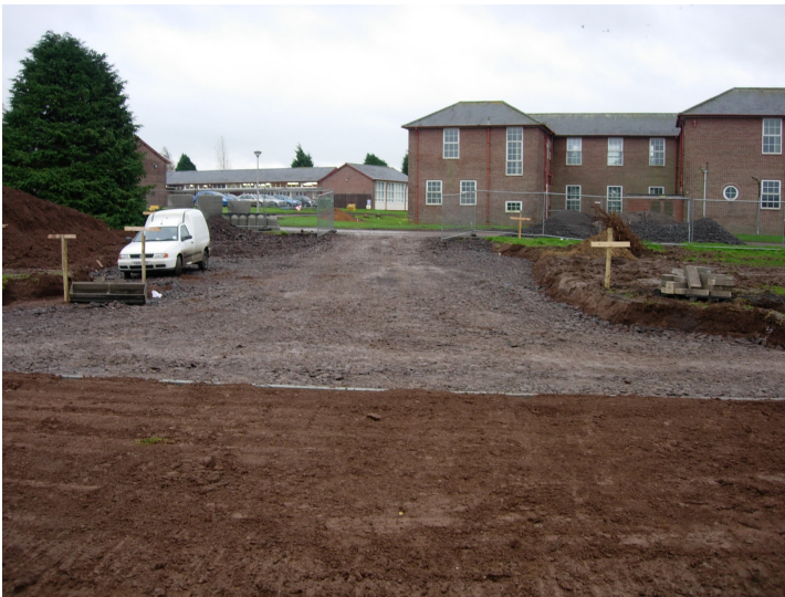
Plate 2 Plant and machinery access laneway (facing south-east).
