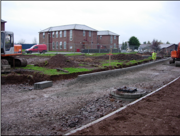
Plate 1 Access laneway running through the site (facing south-west).
