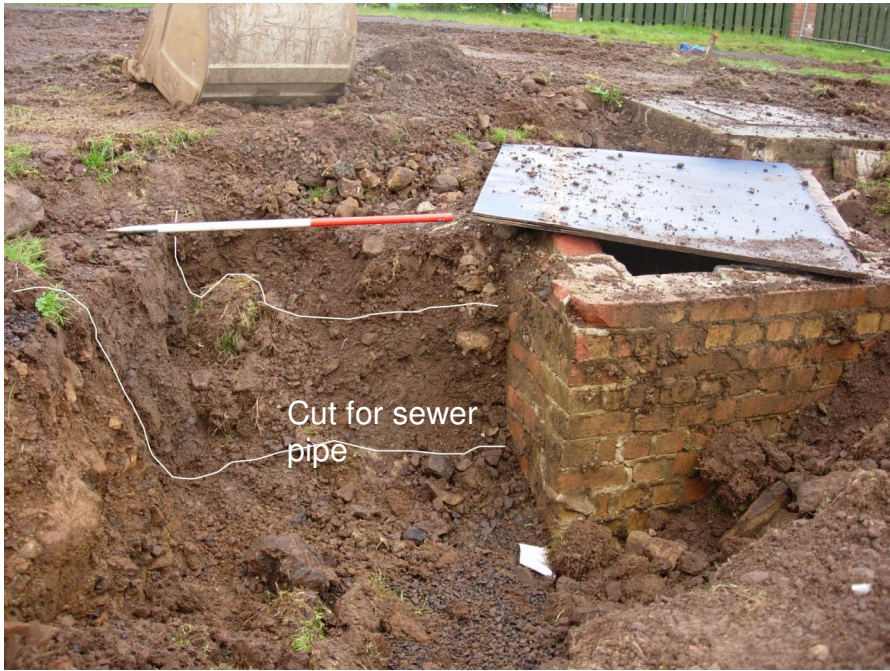
Plate 4. The man hole to the north of the excavated area, showing the cutting and line of the sewer pipe. This was probably a continuation of the feature (context 103) exposed in the excavated area.
