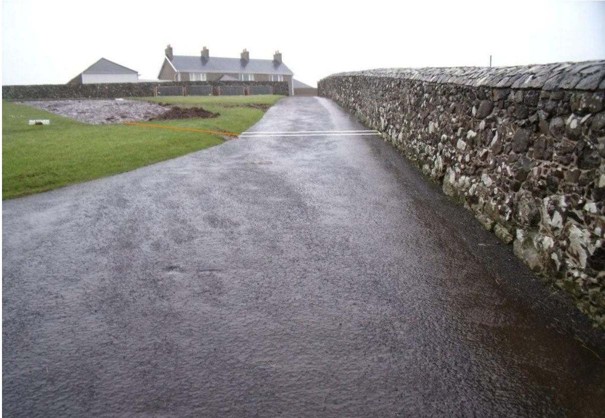
Plate 7 The orange line indicates the line and direction of the drainage pipe sited below ground level to displace storm water from the dig to the precast drain. The white line indicates the position of the precast drain across the tarmac lane (pre-excavation photo).
