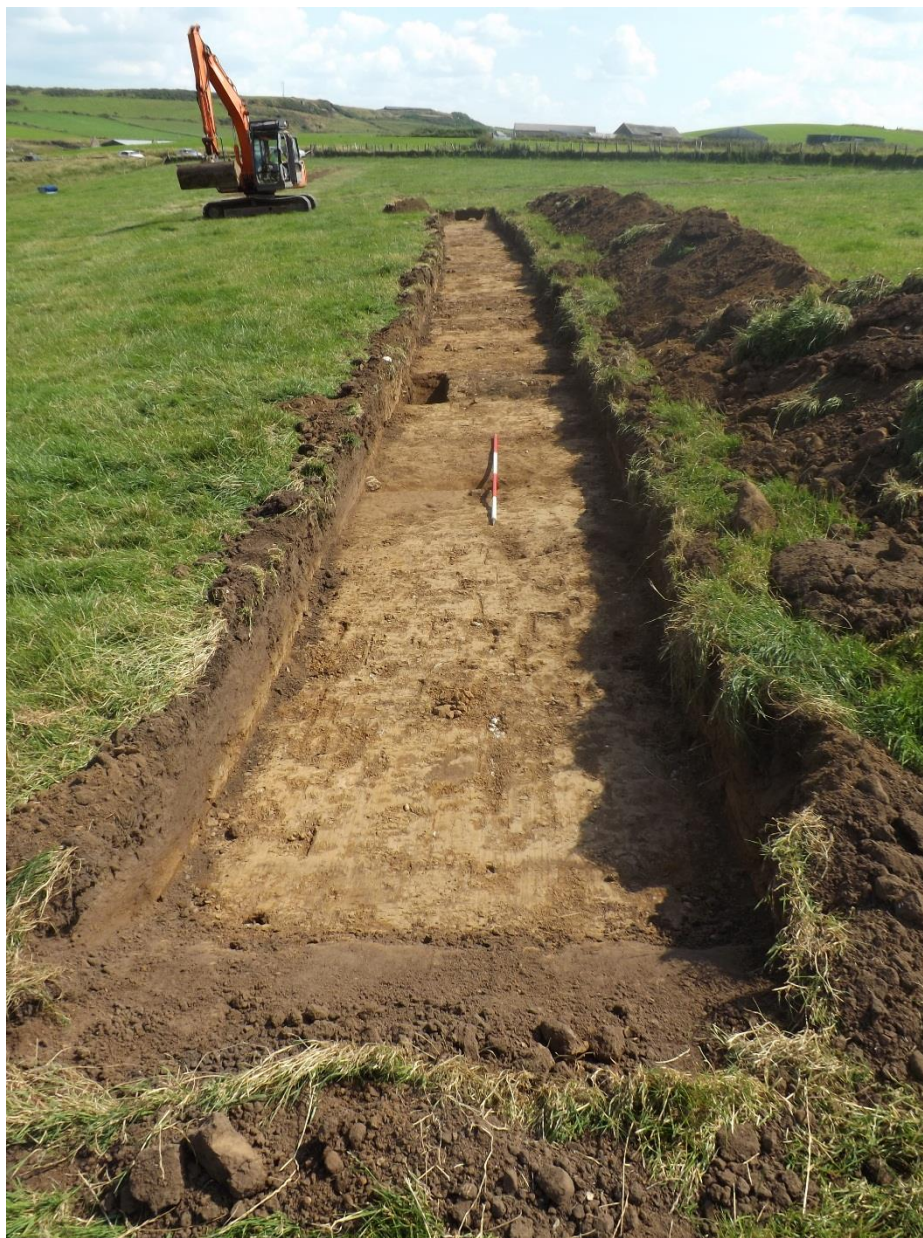
Plate 20: Trench 16, following excavation, looking South-East
