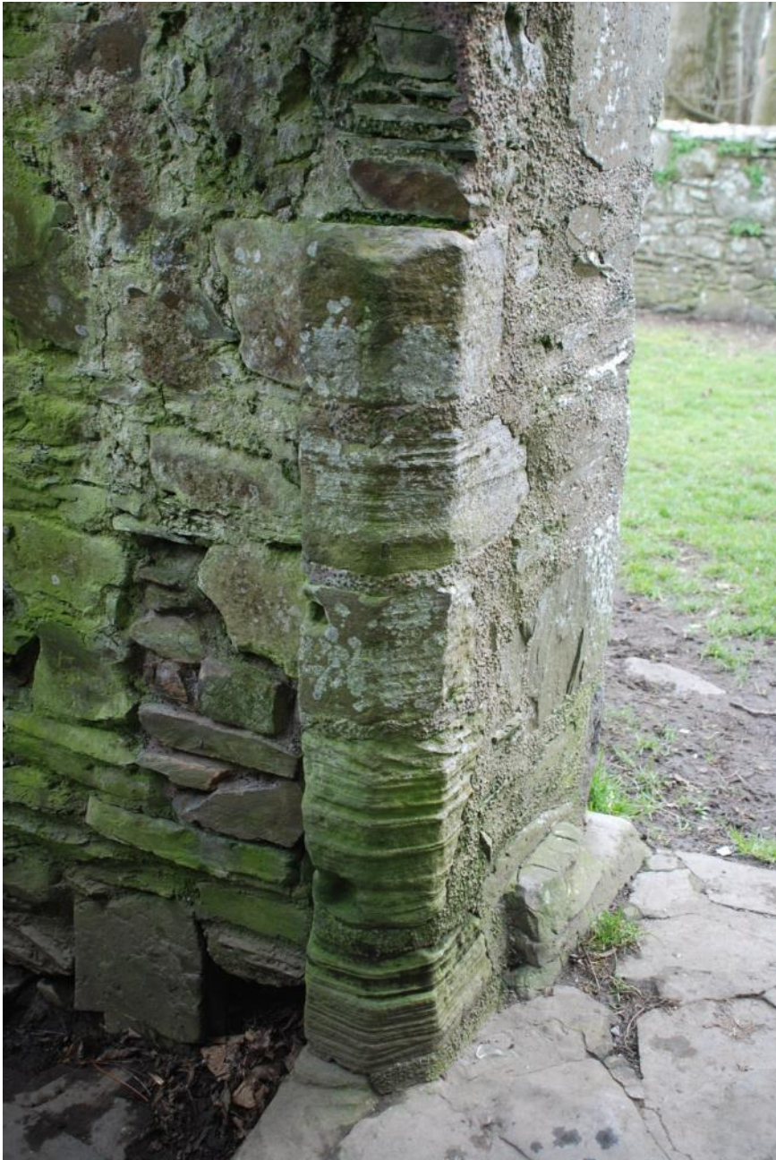
Plate 62 Carved sandstone door mouldings in the women's bathhouse at Struell (photo F. McCormick, QUB).
