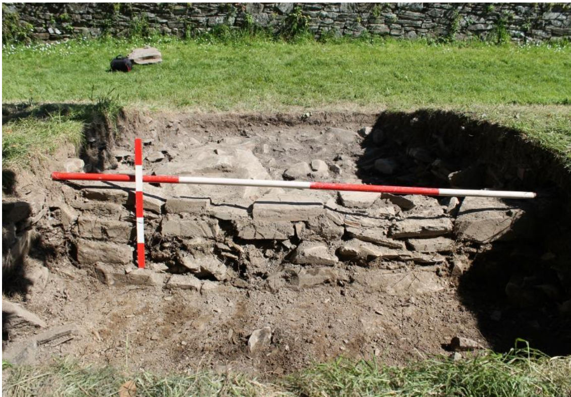
Plate 51 The west face of wall C603, looking east
