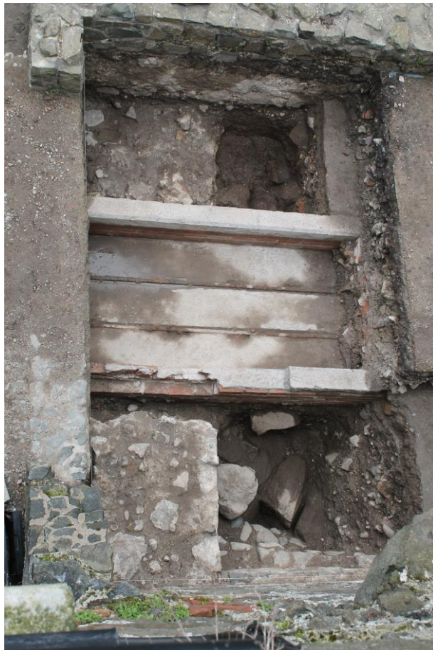
Plate 15. Inner Ward. Trench 1. The Medieval wall C.106/C.135 crossed by the Victorian railway. From east.
