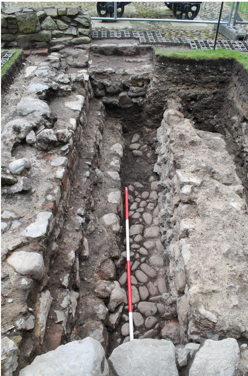
Plate 42. Outer Ward. Trenches 5 and 8. Wall C.512, cobbles C.819, the southern gable and footings of the barracks building (C.809 and C.818) and the junction with the above-ground east wall of the building. From west.
