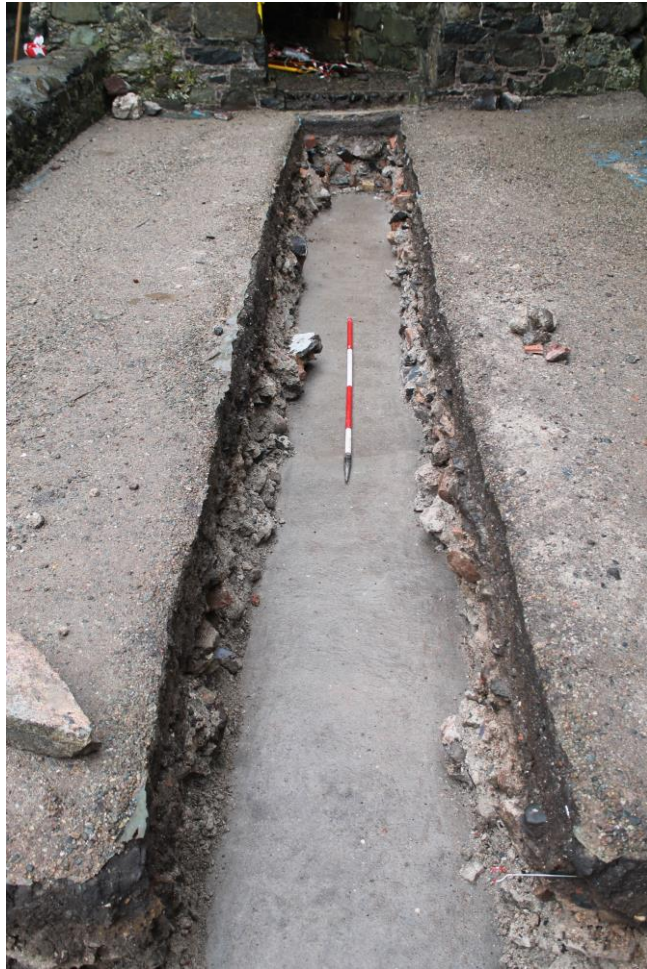
Plate 17. Inner Ward. Trench 2. Demolition layers and concrete surface C. 210. From south.
