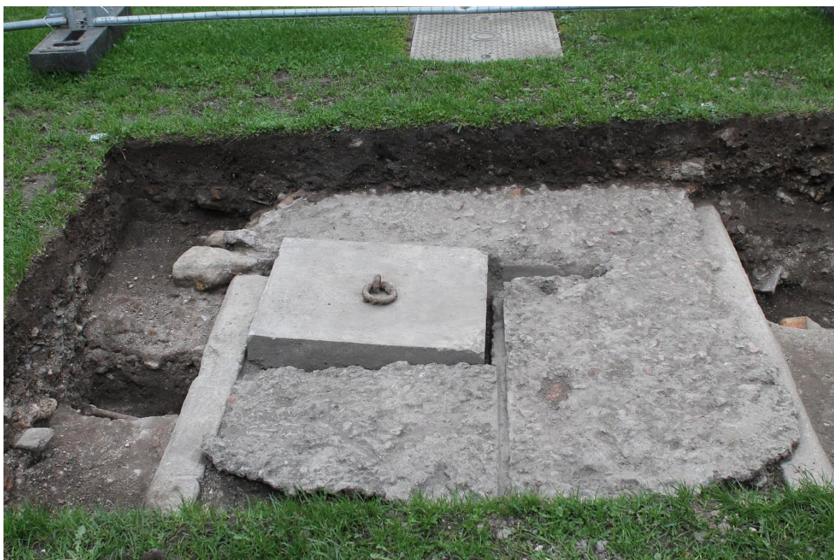
Plate 33. Inner Ward. Trench 4. The visible granite sleepers of the Victorian railway and the later manhole cover. From east.
