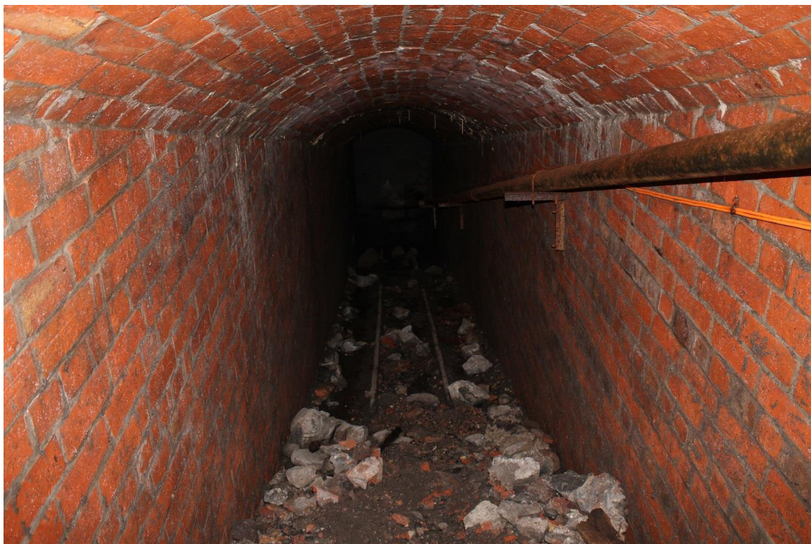
Plate 35. Inner Ward. The still extant subterranean Victorian railway as seen after being accessed from the manhole cover adjacent/ west of Trench 4. Looking west down the railway tunnel.
