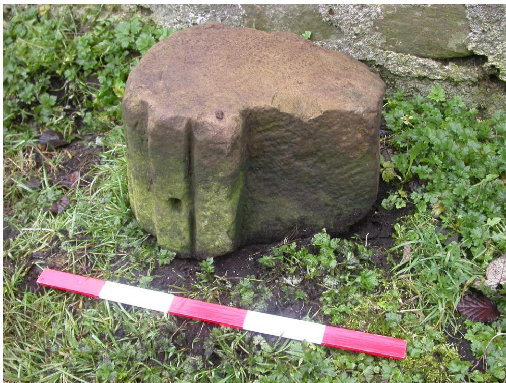
Plate Two: Window jamb within the graveyard at St Patrick’s Eglisish (Roan). Note the glazing groove and adjacent socket for a horizontal bar. Broadly dated to AD 1200-1600. Scale 0.50 metres.
