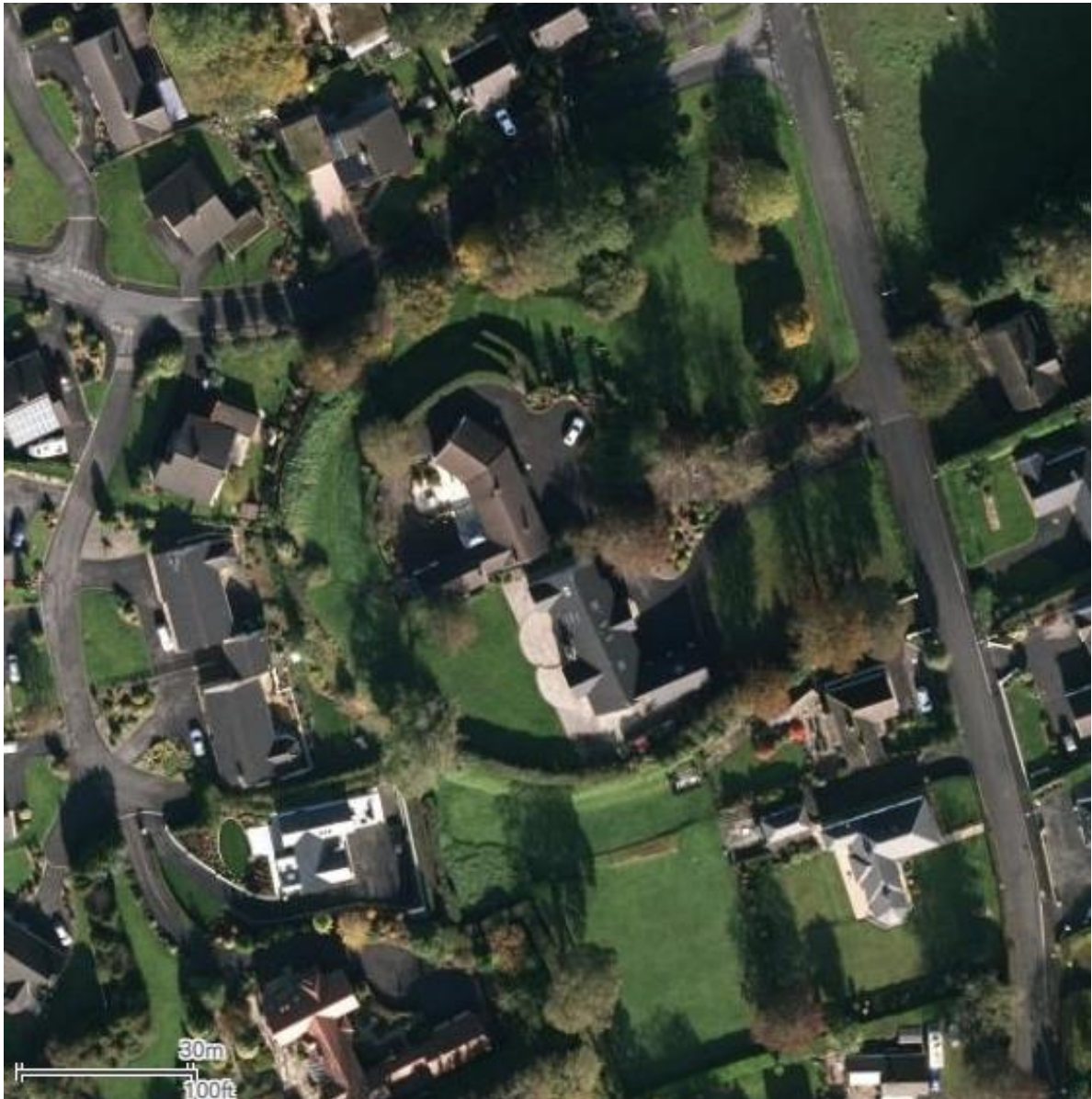
Plate 2. Detailed aerial photograph showing the location of Lisdoon bivallate rath and the modern buildings within the interior of the monument, Lisnaskea village, County Fermanagh. From the HED Historic Environment Map Viewer (accessed August 2022).
