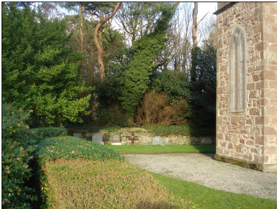
Figure 11: View of church wall and mound, looking north
