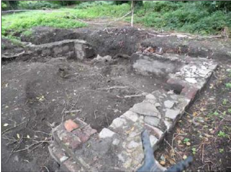
Pl 1: View of exposed northwest corner wall foundations. (M. Conway, NT)
