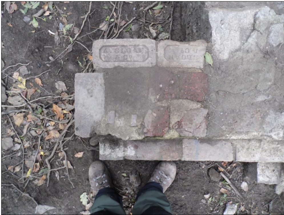
Pl.7: Detail top of brick pier, east end of wall W1, showing bricks by 'A. Sloan & Co.' (M. Conway, NT)
