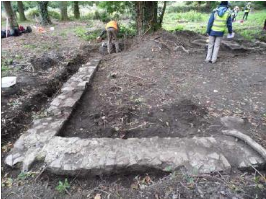
Pl 3: View from north of the east side of the North compartment showing tree roots covering the line of the south wall (W4), (M. Conway, NT)
