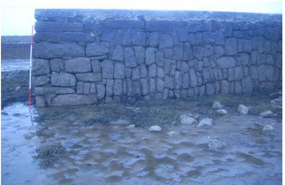
Plate 42: Ringneill Quay. North face, eastern end.
