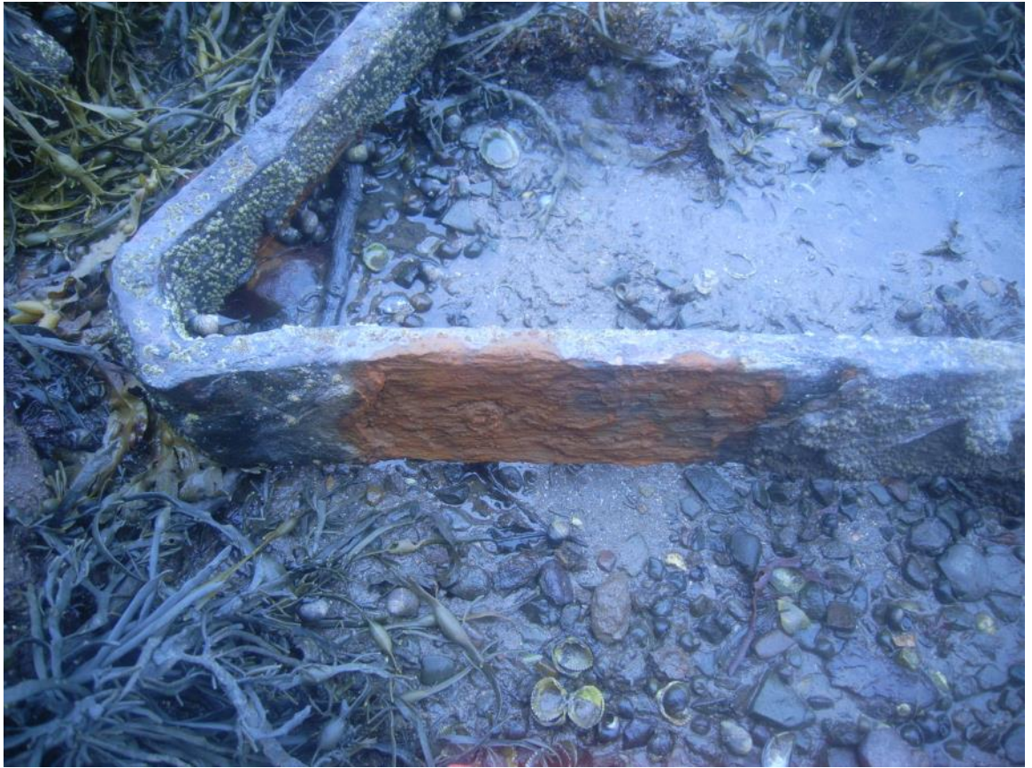
Plate 23: Detail of iron bracing component.
