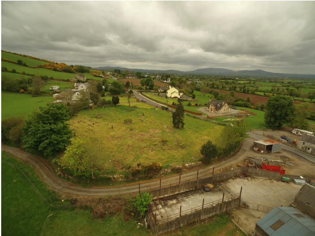
Figure 2: Aerial View of the site looking South.
