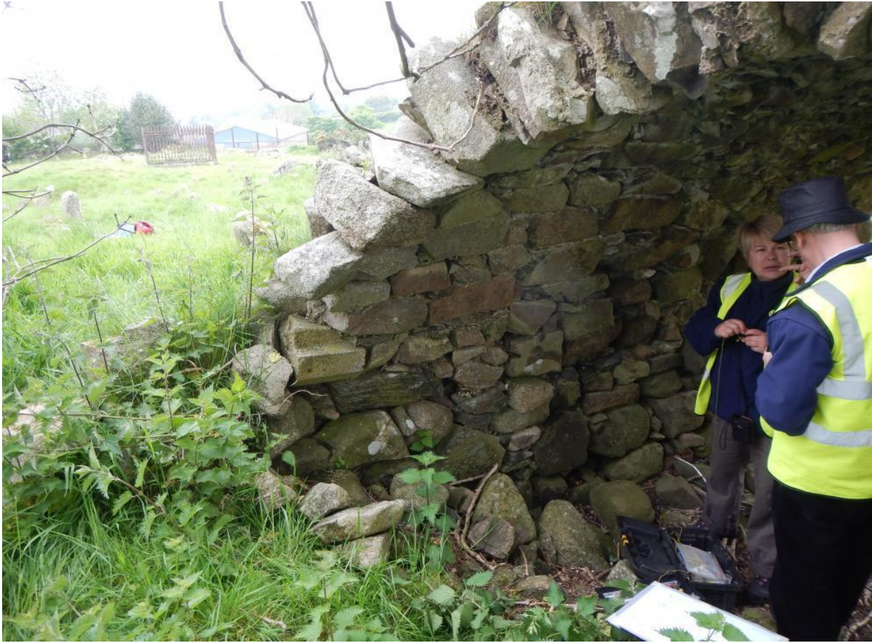
Figure 14: Members of the Survey Team examining re-used dressed stone.
