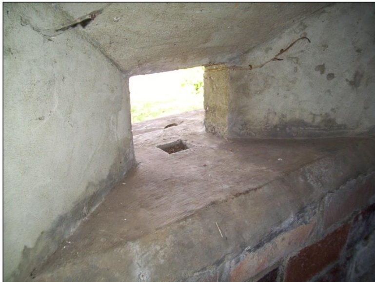
Figure 15: Inside a Type 22 Pillbox in Elstead, Surrey, complete with concrete loop-hole tables, www.pillbox-study-group.org.uk
