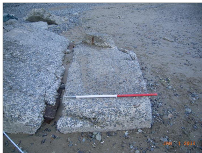
Figure 27: Metal rails used as roof supports
