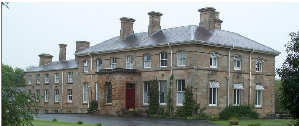
Figure 23: Murlough House, Dundrum, County Down, Courtesy of Andy Glenfield, The Second World War in Northern Ireland at www.ww2ni.webs.com
