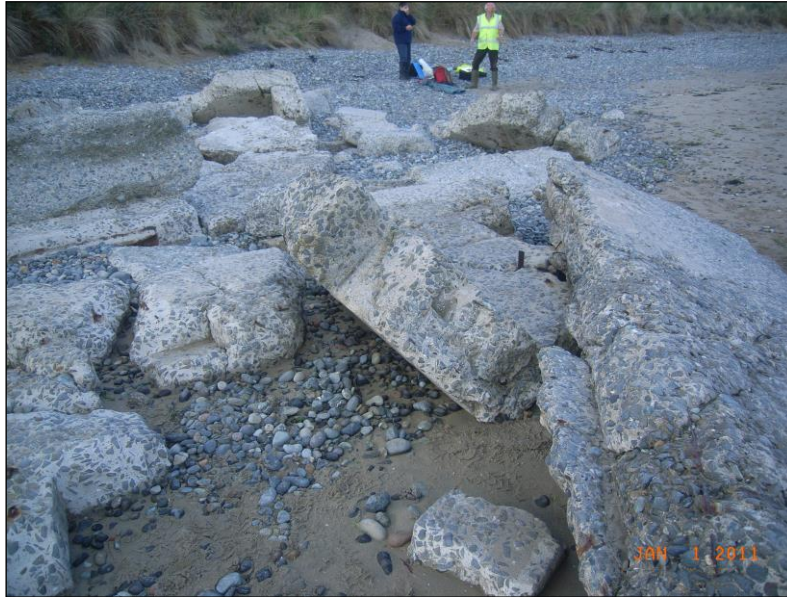
Figure 30: Angular stones set into concrete matrix
