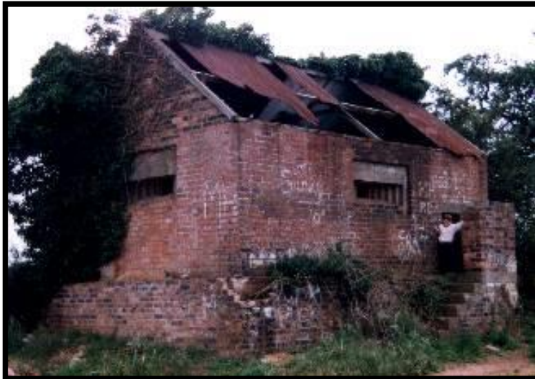
Figure 13: Large Pillbox at High Ercall, Shropshire, disguised as a house, www.pillbox-study-group.org.uk
