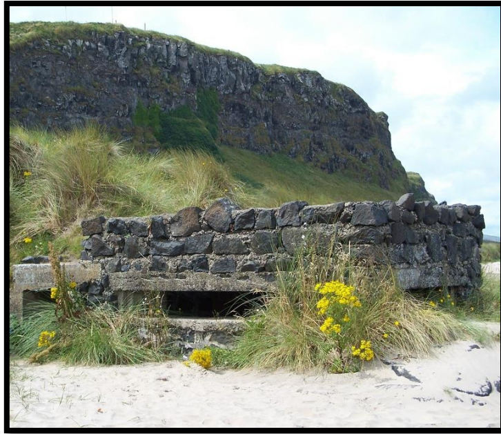
Figure 18: Downhill Pillbox, with basalt blocks as additional camouflage Courtesy of Andy Glenfield, The Second World War in Northern Ireland at www.ww2ni.webs.com
