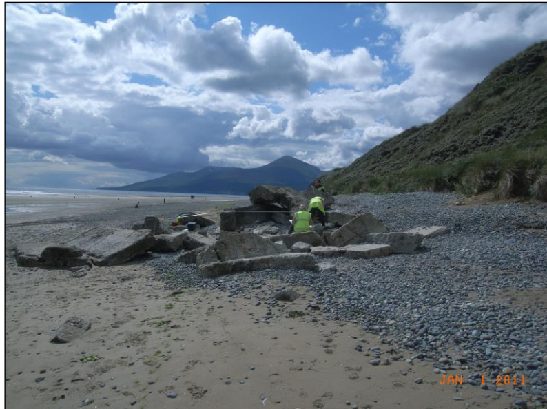
Figure 7: View of Pillbox remains, with Mourne Mountains to the south
