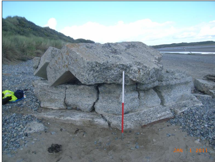
Figure 26: Evidence for sectional construction
