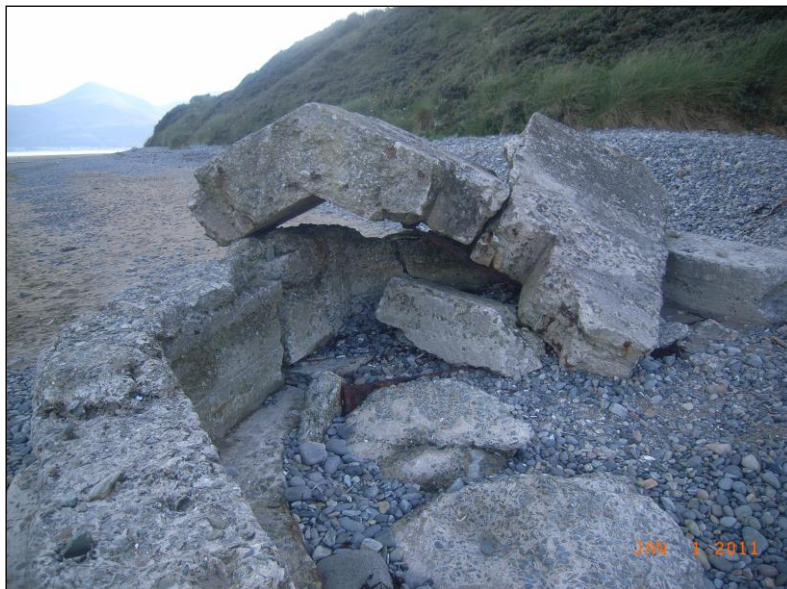
Figure 31: Iron/metal items within the Pillbox structure
